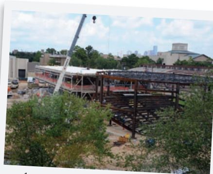
Auditorium beginning to take shape August 2009
