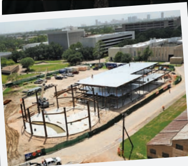
Framing up! July 2009
