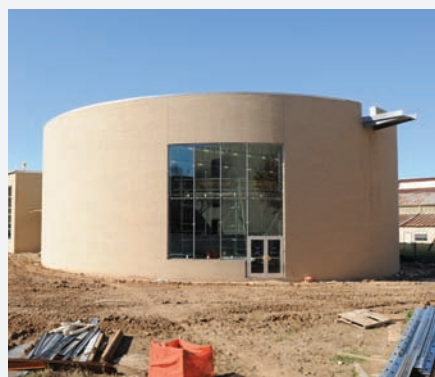
February 2010 Exterior is done and glass is too.
